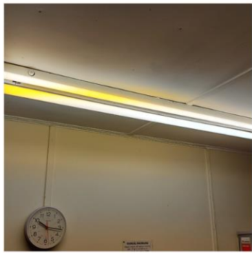
E213: Lighting appears reduced light output, diffuser missing.
