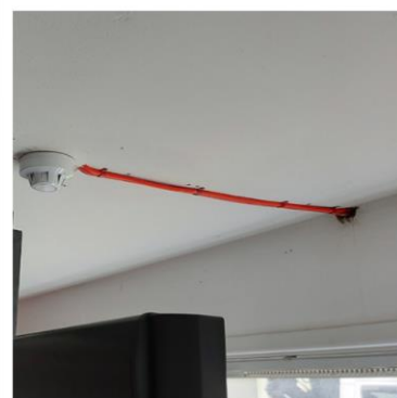
E209: Fire alarm detector heads – recommend repositioning.
