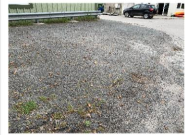
B109: Tarmacadam to the front and sides of the building are worn and breaking up
