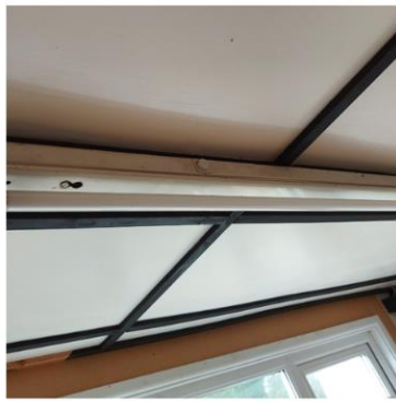
E214: Light fitting diffuser missing.
