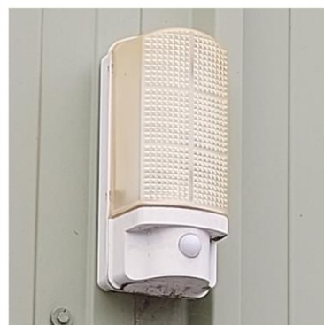
E221: External lighting degraded diffuser.
