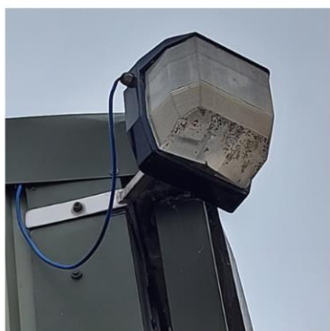
E219: External lighting with signs of water ingress.
