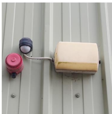
E217: External lighting degraded diffuser and PIR detector.
