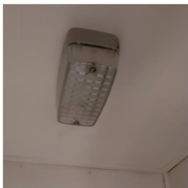
E216: Bulkhead fitting not working.
