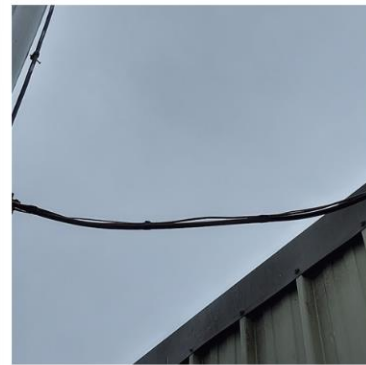
E206: External cables to be supported
