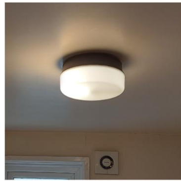
E215: Circular surface downlight, reduced light output.
