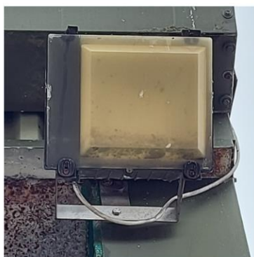
E220: External lighting degraded diffuser and internal algae growth.
