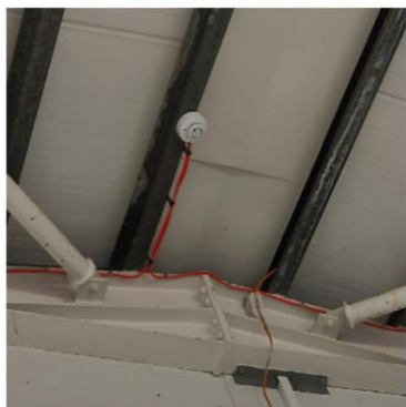
E210: Fire alarm detector heads – recommend repositioning.
