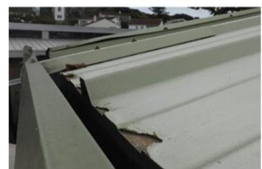
B112: Cut edge corrosion to the corrugated panel roof
