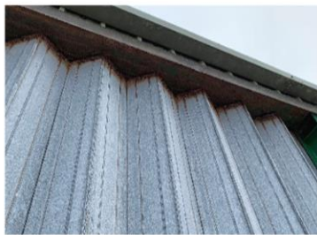
B107: Corrosion to the top and bottom of all 3No. Shutters / Corrosion to the door frames and reveal
