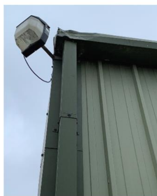
B111: Impact damage to 2No. Panel, Corroded rivets to cladding sheets
