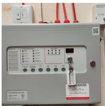
E207: Fire alarm panel in good condition.
